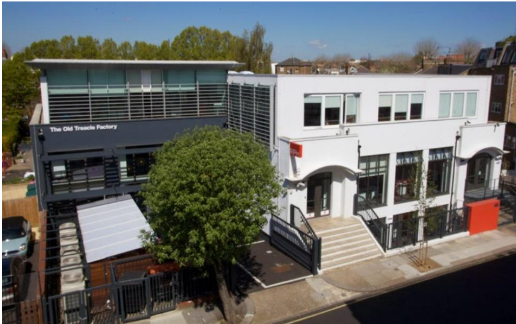
Old Treacle Factory, Goodwin Road - existing
