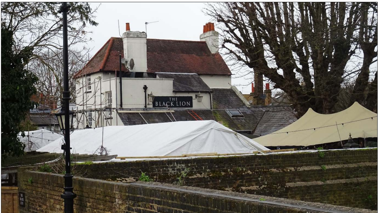
Eradication of open garden setting, alien, poor quality structures.
