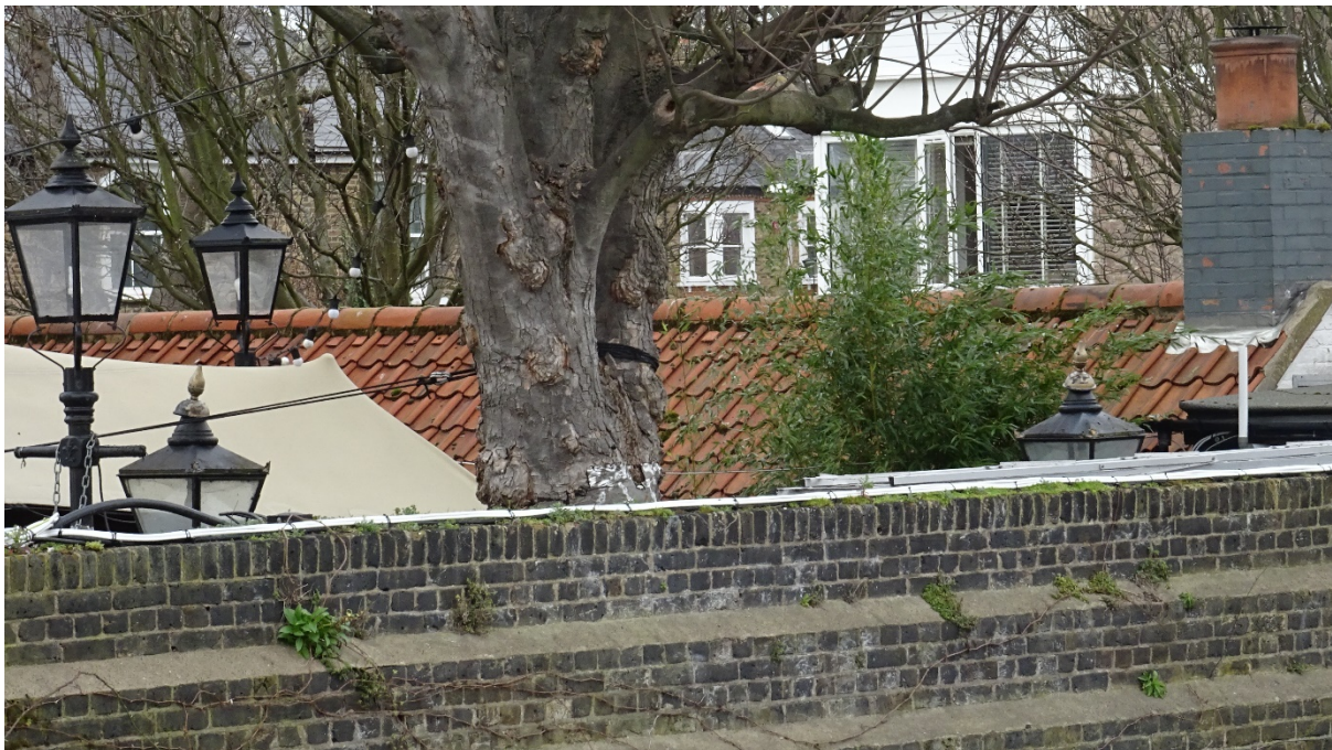
Tent and unauthorised timber structures adjacent to listed Skittle Alley
