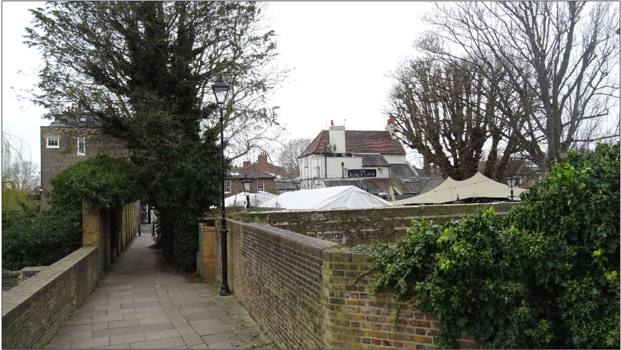
Harm to setting of pub, other listed and locally listed buildings from Thames Path
