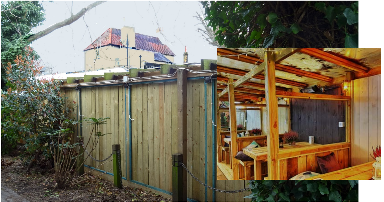
S boundary, open setting/view from Thames Path, (see remains of chain bollards) impeded Note alien materials, exposed/vulnerable electrical wiring. Inset- internal view
