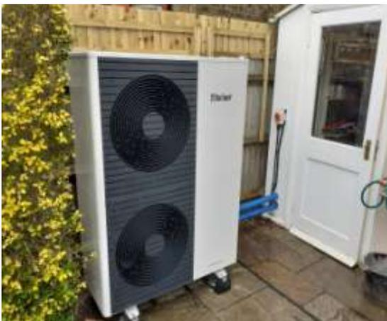
Although tall at 1.5m it is not deep, a mere 45cm and would therefore not protrude far into the garden from the fence but most importantly it has very low noise levels 54db is quoted and only 60db when running flat out.
